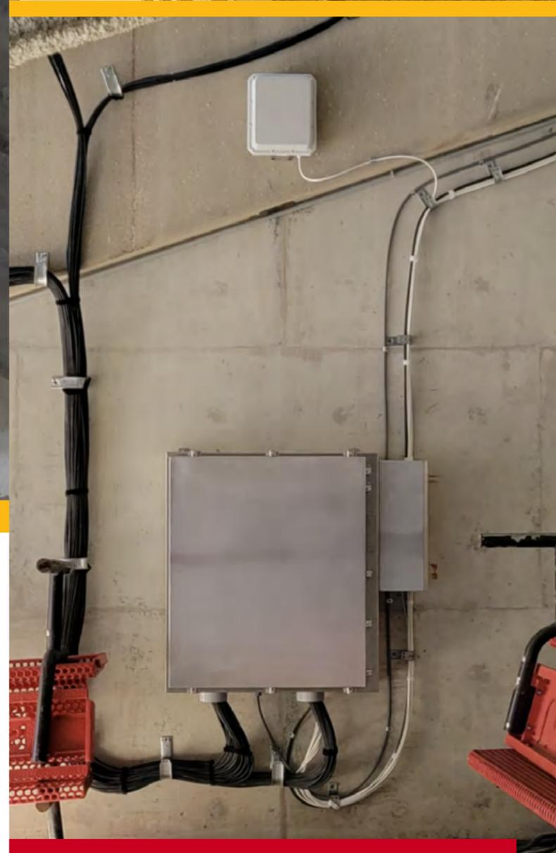
Top: Classic top-down deployments were used where overhangs provided mounting spaces. Bottom: Small IDFs in the concourses connected the seating network to fiber
