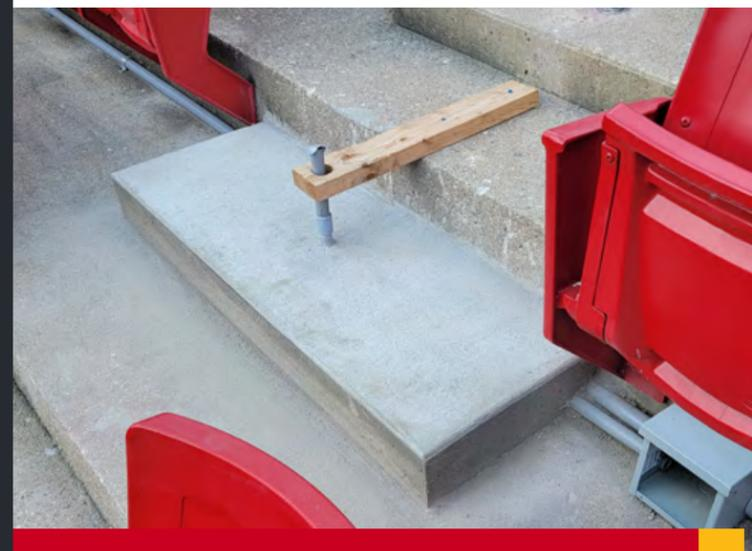
How it started, how it's going: A visual look at the process of demolition and concrete pouring to bring the Wi-Fi conduit to the seats.
