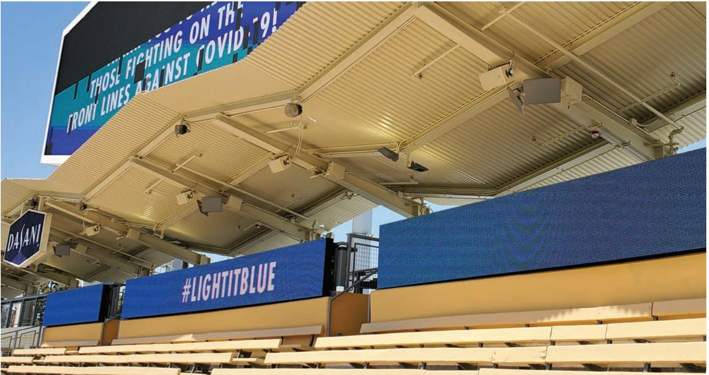
**NEW WI-FI 6 ANTENNAS WERE PLACED IN THE OUTFIELD ROOFS FOR EXPANDED COVERAGE.
