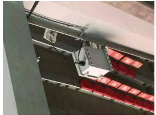
**CLOCKWISE FROM TOP LEFT: WI-FI ABOVE A CONCESSION STAND; A MONITOR TELLS FANS HOW TO LOG ON; AN OVERHEAD LOOK AT AN AP WITH TWIN ANTENNAS POINTING DOWN TOWARD SEATS IN THE B DECK.**
